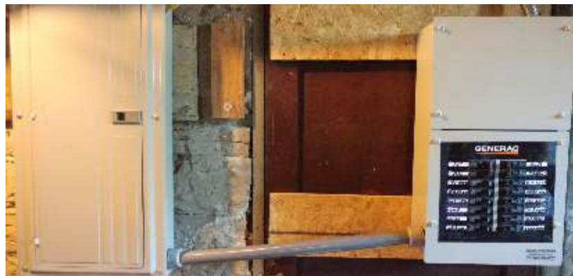
Original house electrical panel on the left, added Transfer panel on the right.
