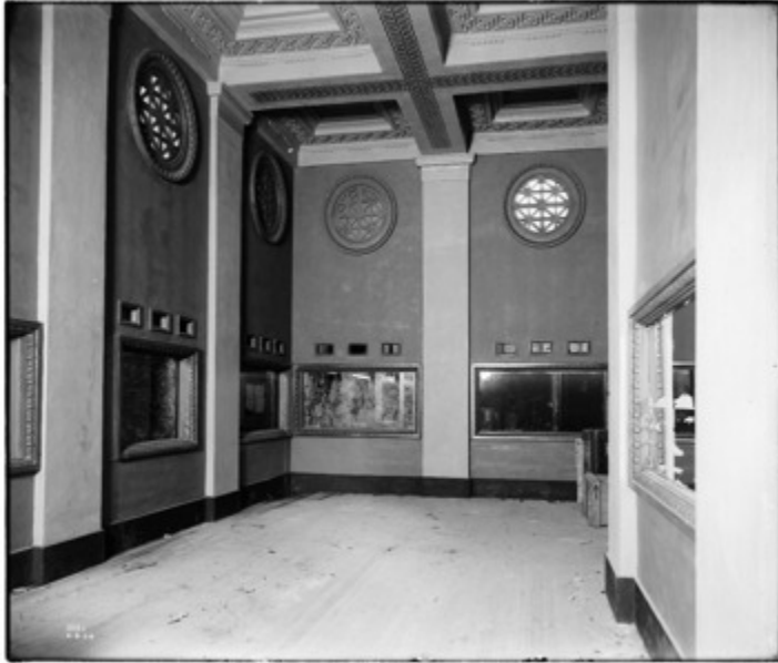
Historical photograph of an aquarium grotto under construction in the Palace of Forestry, Fish, and Game.
